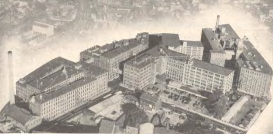
Main Plant, Stanley Tools, New Britain, Conn.
